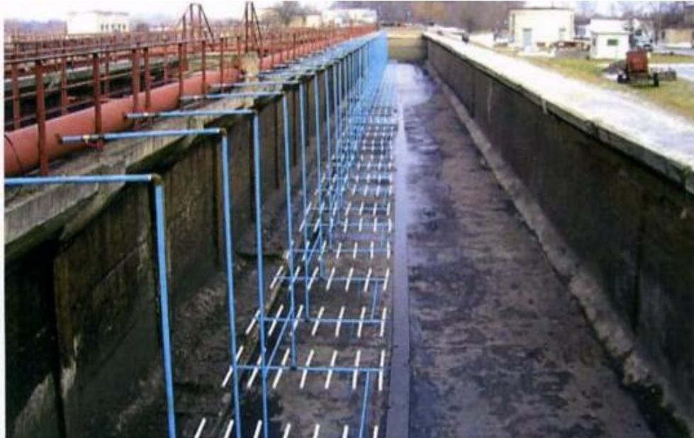
**a) coarse bubble aeration installation at Brest treatment plant**
